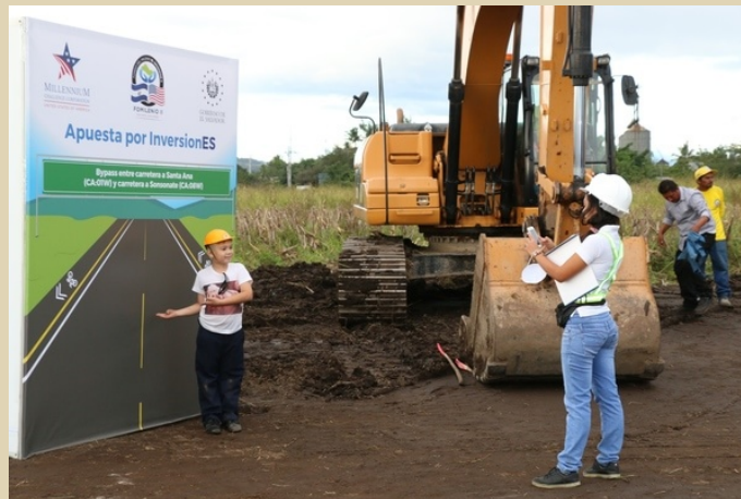
Site of the future Santa Ana - Sonsonante bypass, 2019. Photo courtesy of FOMILENIO II.
